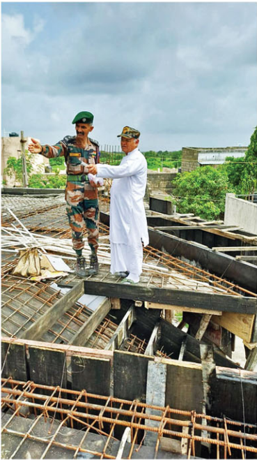
Purusharth Bhojashalaa Ongoing Construction
